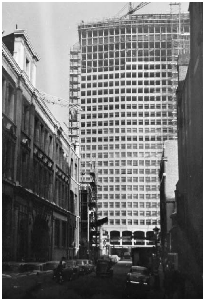
Figure 41 : Stag Brewery and Portland House during Construction (DCA, 2013)
