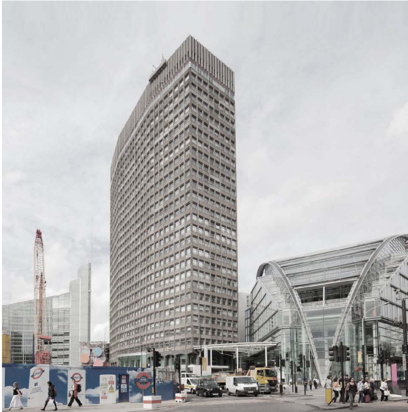
Figure 33 : Portland House, South Elevation - Existing (DCA, 2013)
