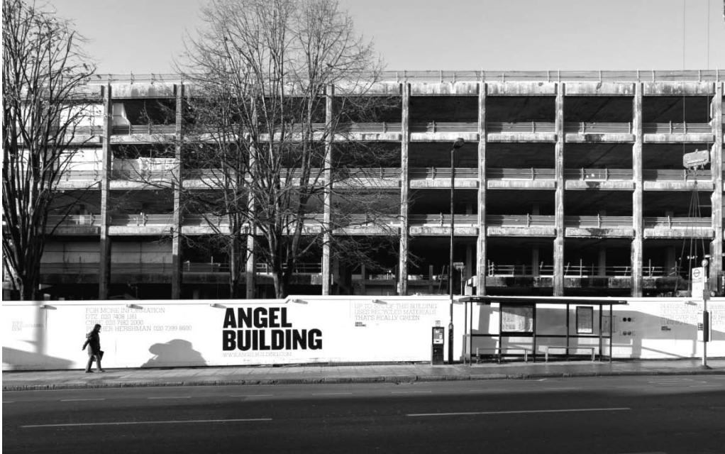
Figure 23 : Angel Building (1980s), during refurbishment (2010). Source: AHMM Architects
