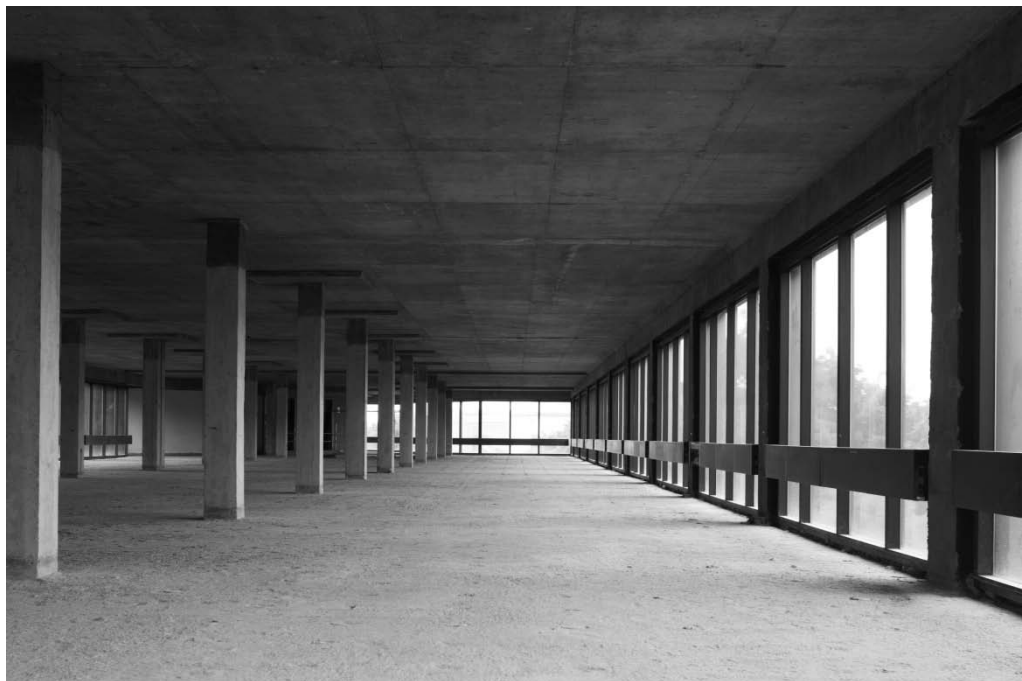
Figure 24 : Angel Building (1980s), during refurbishment (2010) Source: AHMM Architects
