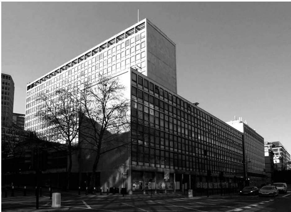
Figure 22 : Fleet Building, to be demolished (2015), Source : LMA
