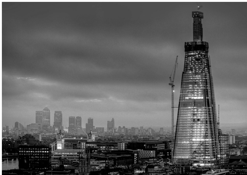
Figure 8 : The Shard during construction, 2013. Source, The Telegraph.
