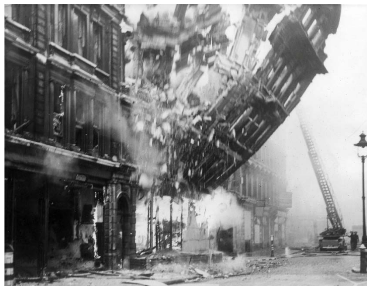
Figure 4 : Demolition of Victorian buildings, Victoria Street (1944) , Source: LMA
