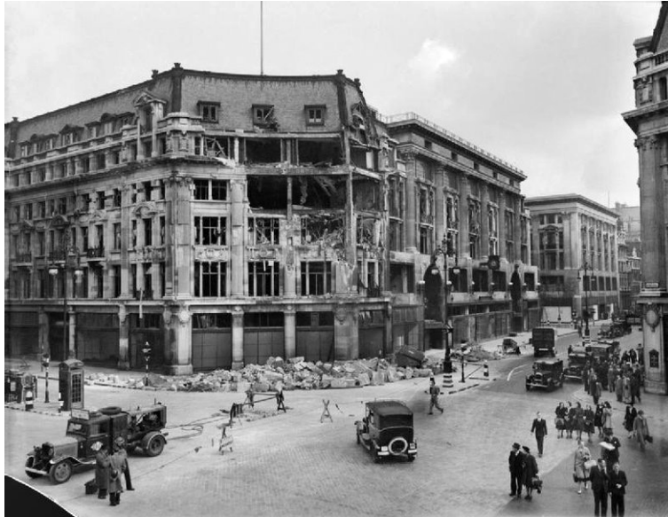
Figure 2 : Offices in Oxford Circus (1940). Source: LMA
